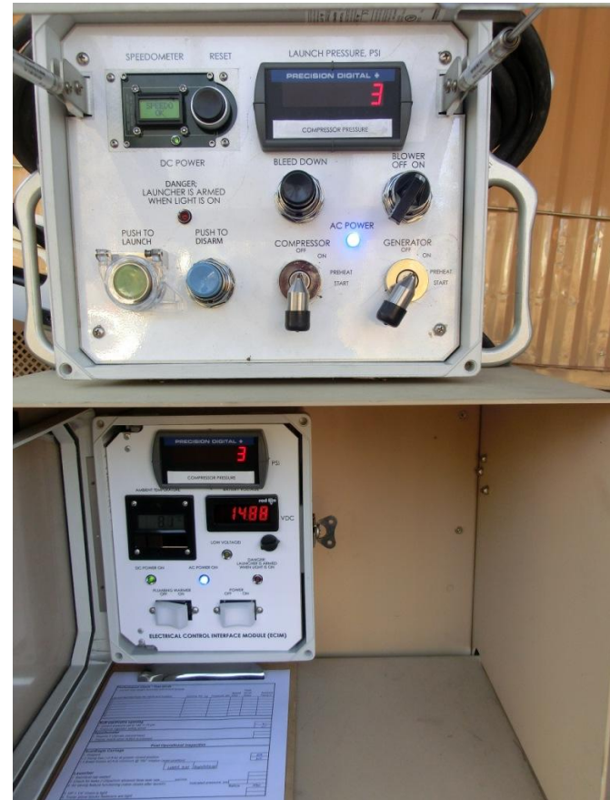
Error Eliminator Installed
